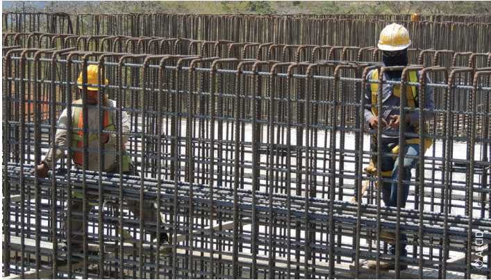
Work progress at waste water treatment plant in Masaya
